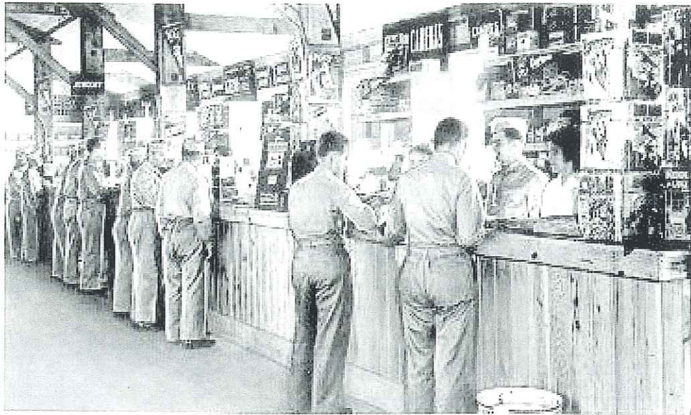
ONE OF THE MANY POST EXCHANGES, CAMP KILMER, N. J.
